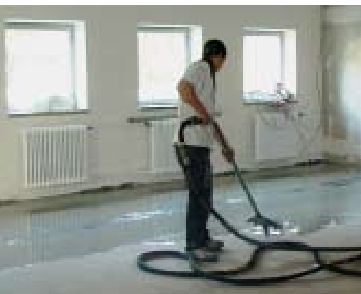
Levelling compound is a self-levelling compound that is used to eliminate any unevenness.
