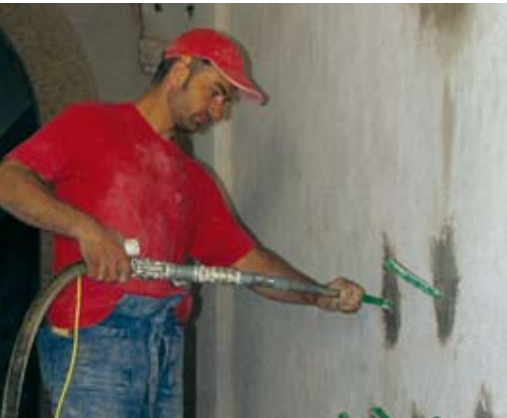
3 The Sprayboy injecting mortar into the holes.
