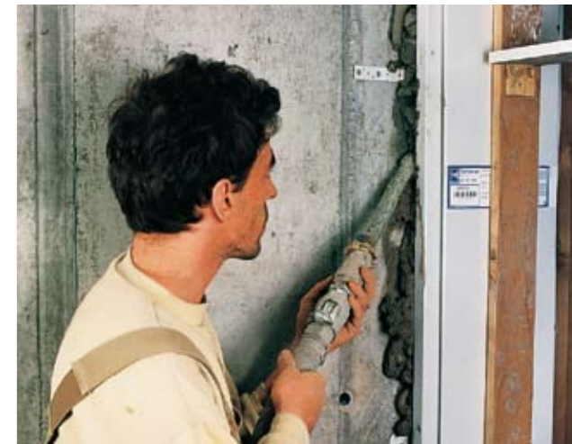
It is the ideal machine for small jobs, such as here for filling door frames or for refurbishment work.
