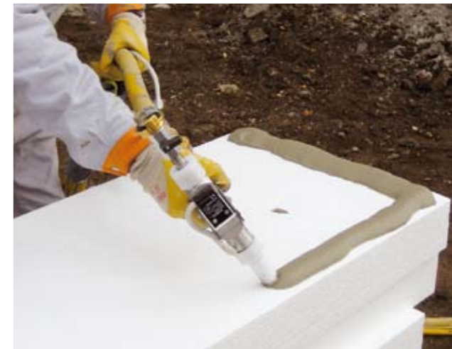
You can use the MP 22 without any problems for more sophisticated operations such as here for heat-insulating material.
