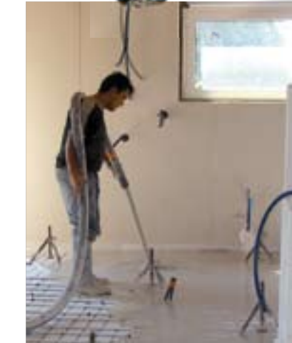
Liquid screed with the S 5 EF
