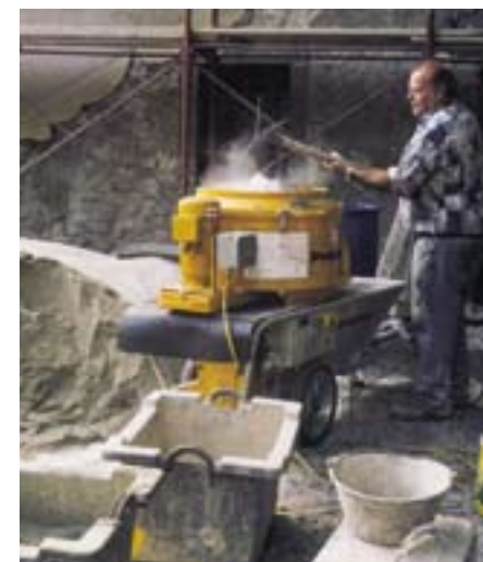
Filling the S 5 EVTM with a shovel
