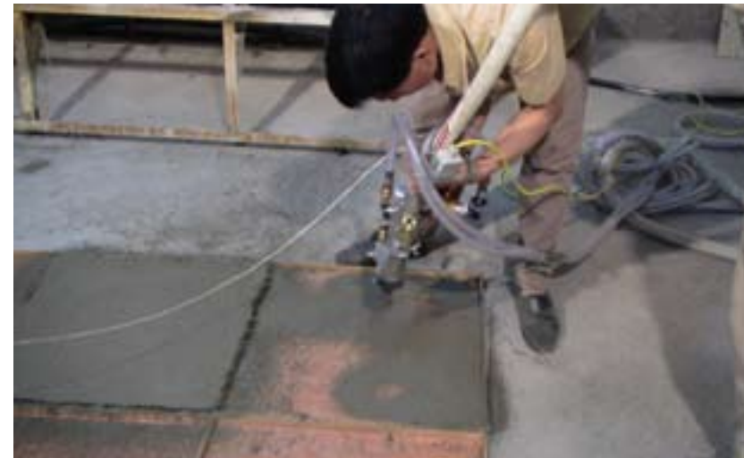
Making fibre-reinforced concrete slabs
