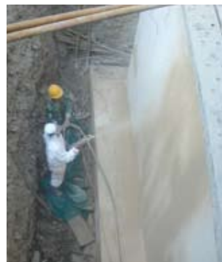
Coating concrete foundations
