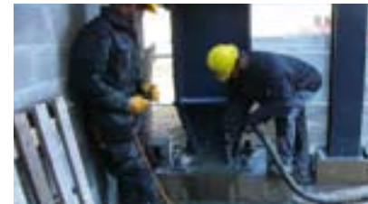
Filling steel columns in a car park
