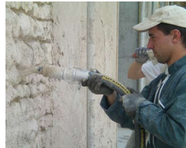
SP 11 worm pumps can be used inside and out for all site-made mixes and premixed dry mortar up to 6 mm.
