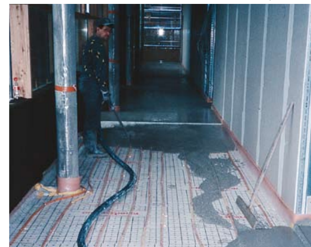
With the appropriate worm parts, you can even pump self levelling floor screed easily and economically.
